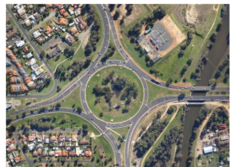
... and after the upgrade.
